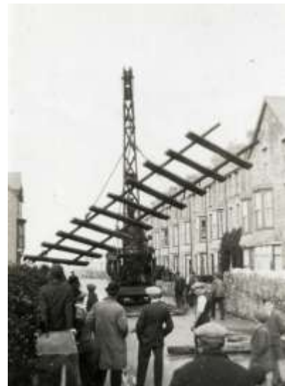
Laying train track in 1930
